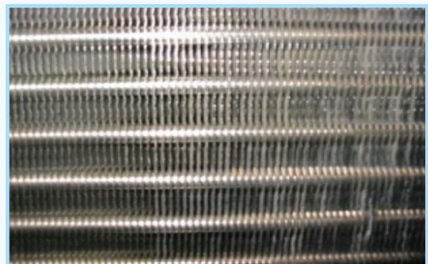
Coil After UV Application
